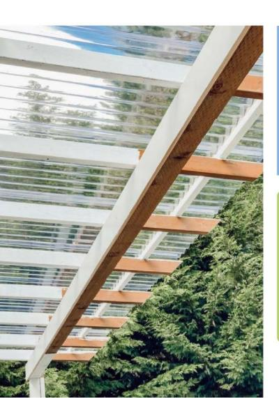
Due to such qualities as a high level of strength and transparency, wave polycarbonate is widely used in industrial, commercial and agricultural constructions.
