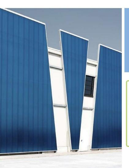
Multiwall polycarbonate interlocking modular systems are an innovative solution for use in architecture in the exterior and interior, where a system of translucent walls is required.
